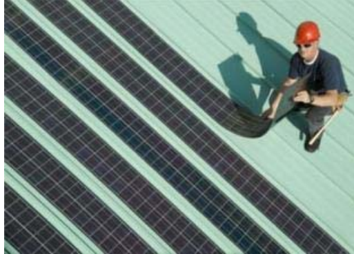
Figure 8 CIS thin-film
